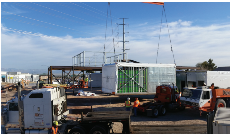
Photo of BLOX construction site
