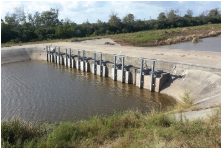
Photo of Jefferson County Drainage Site
